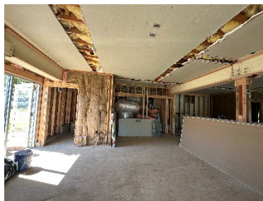
The interior of the St. Maries Public Library building during construction.
